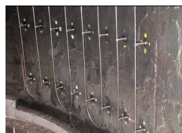
Installation Options SAVELINE® Installation on Spacer Bolts
