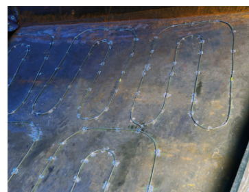
Layout of SAVELINE® sensors at the bottom of the lower vessel
